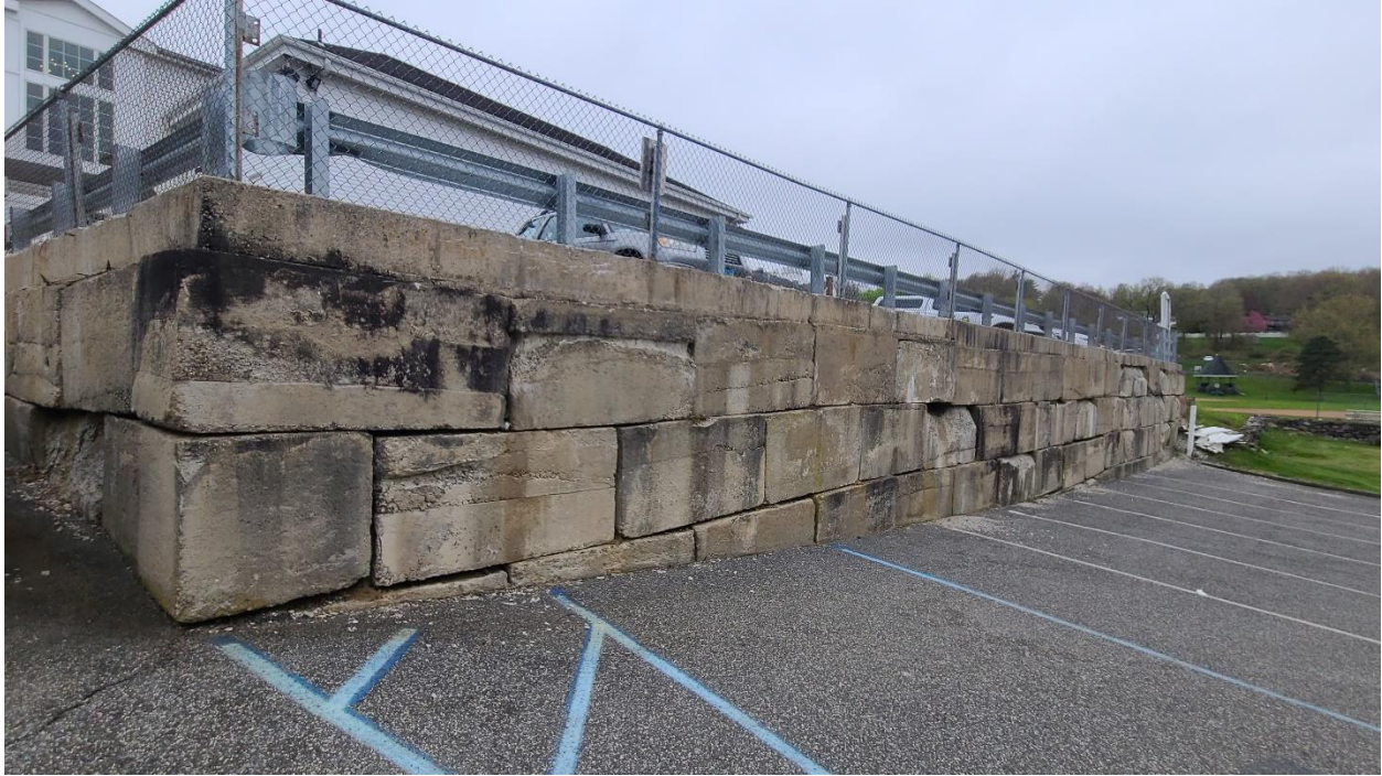
Photograph 3: Parking lot retaining wall
