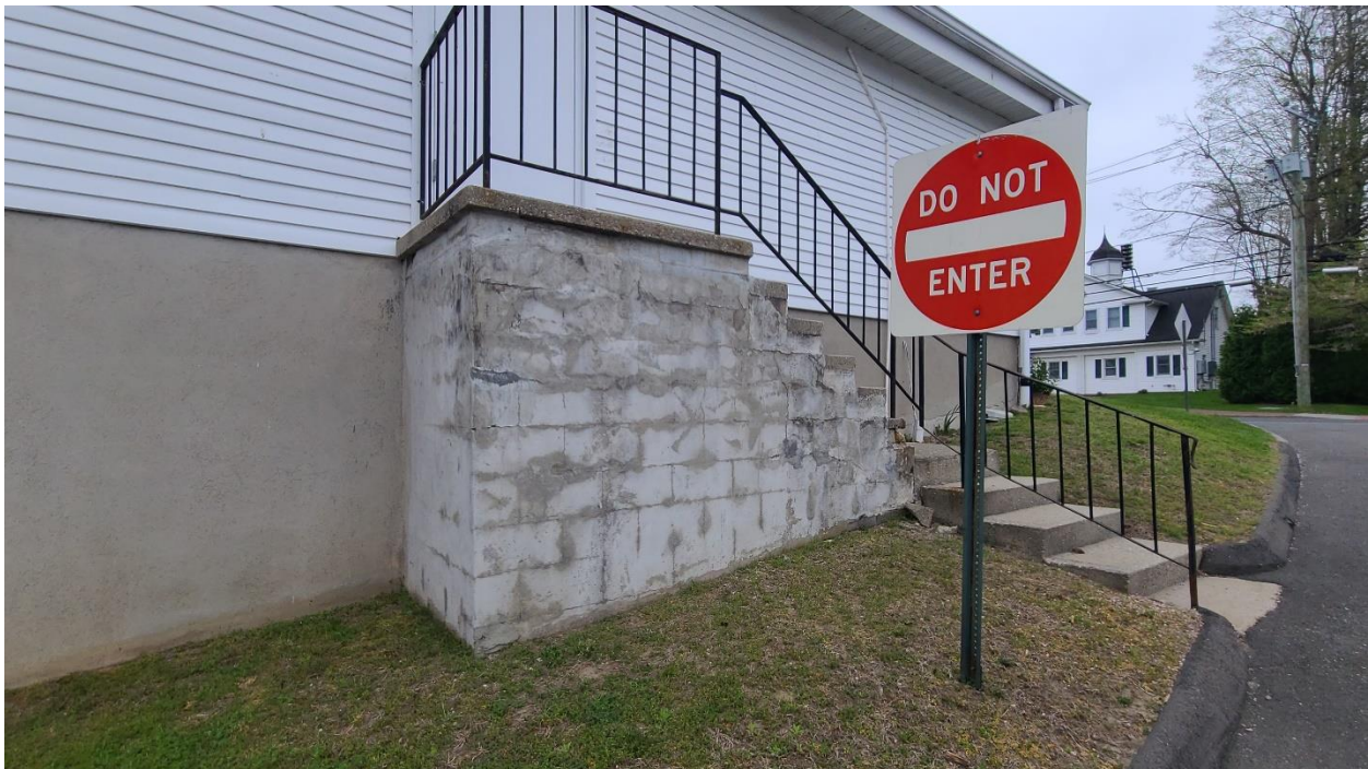
Photograph 2: Emergency egress landing and stairs
