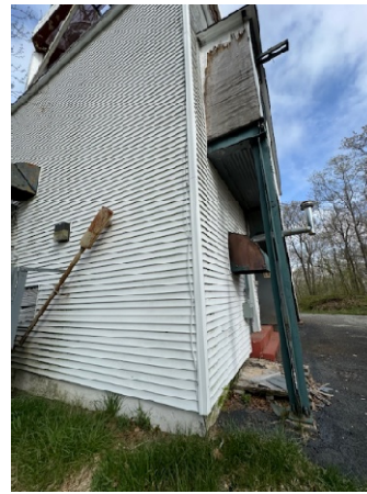
Column supporting exterior stair landing
