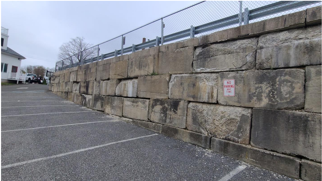
Photograph 4: Parking lot retaining wall
