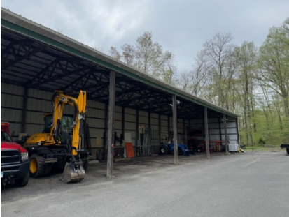
Storage Shed Building
