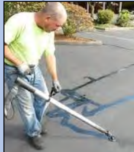
Sealing Roadway Cracks
