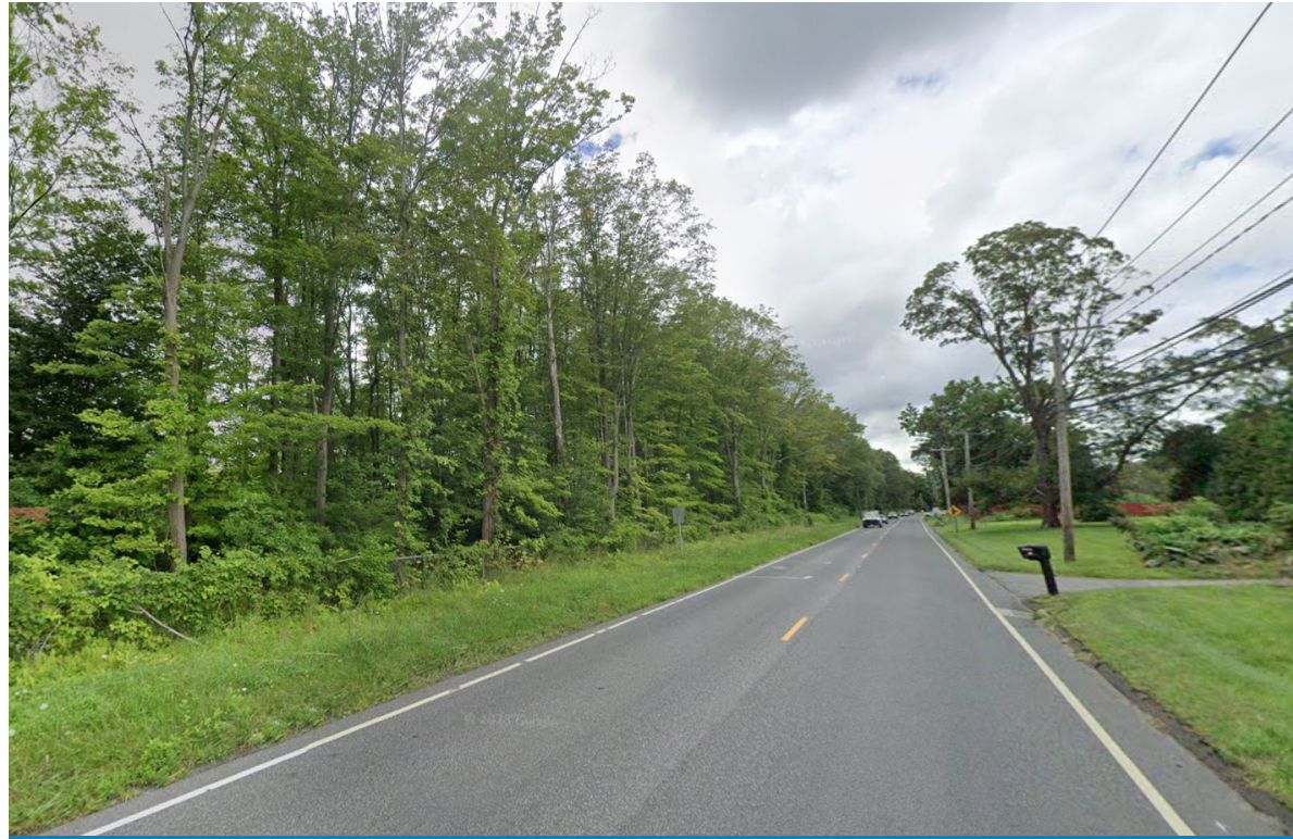
Pembroke Road - Existing Conditions
