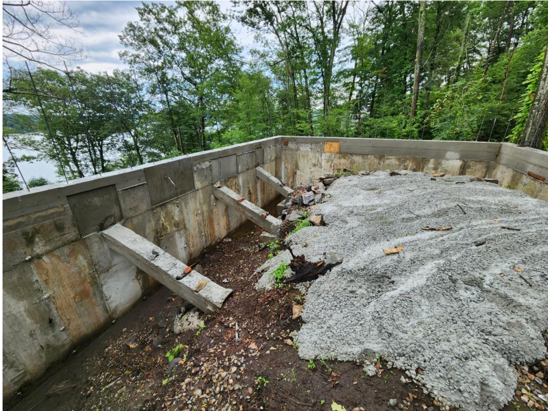
Photograph 2: Overall view of counter forts/butresses.
