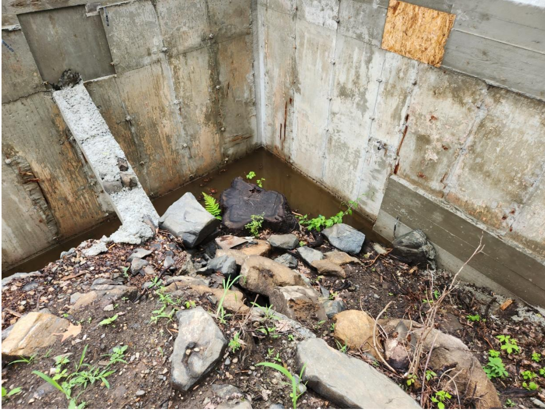
Photograph 4: Observed tree trunk/roots in excavation.
