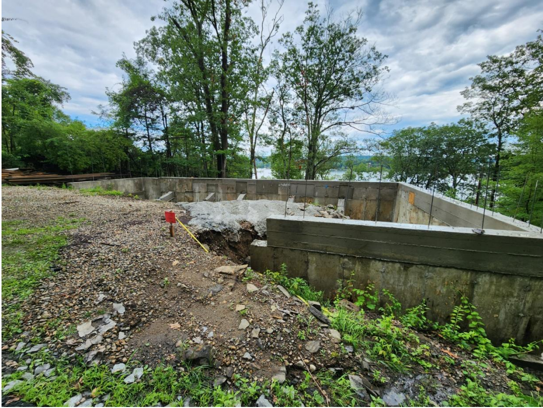
Photograph 1: Overall view of parking structure.
