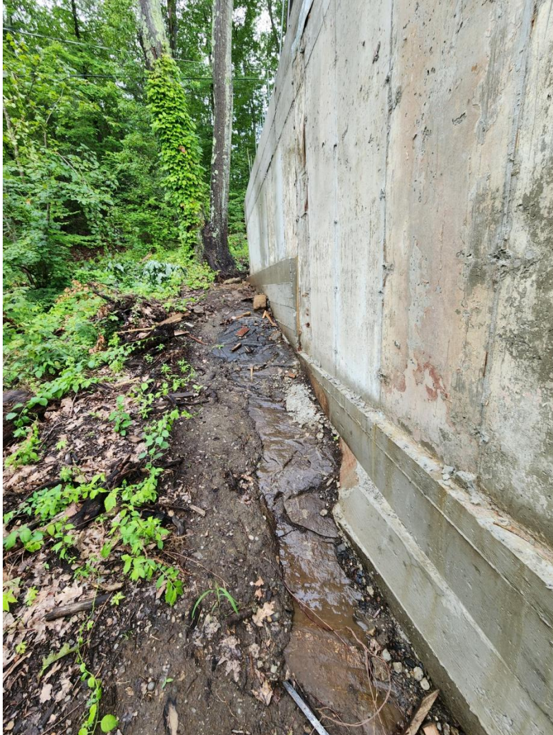
Photograph 3: Bedrock observed at stem wall casting.
