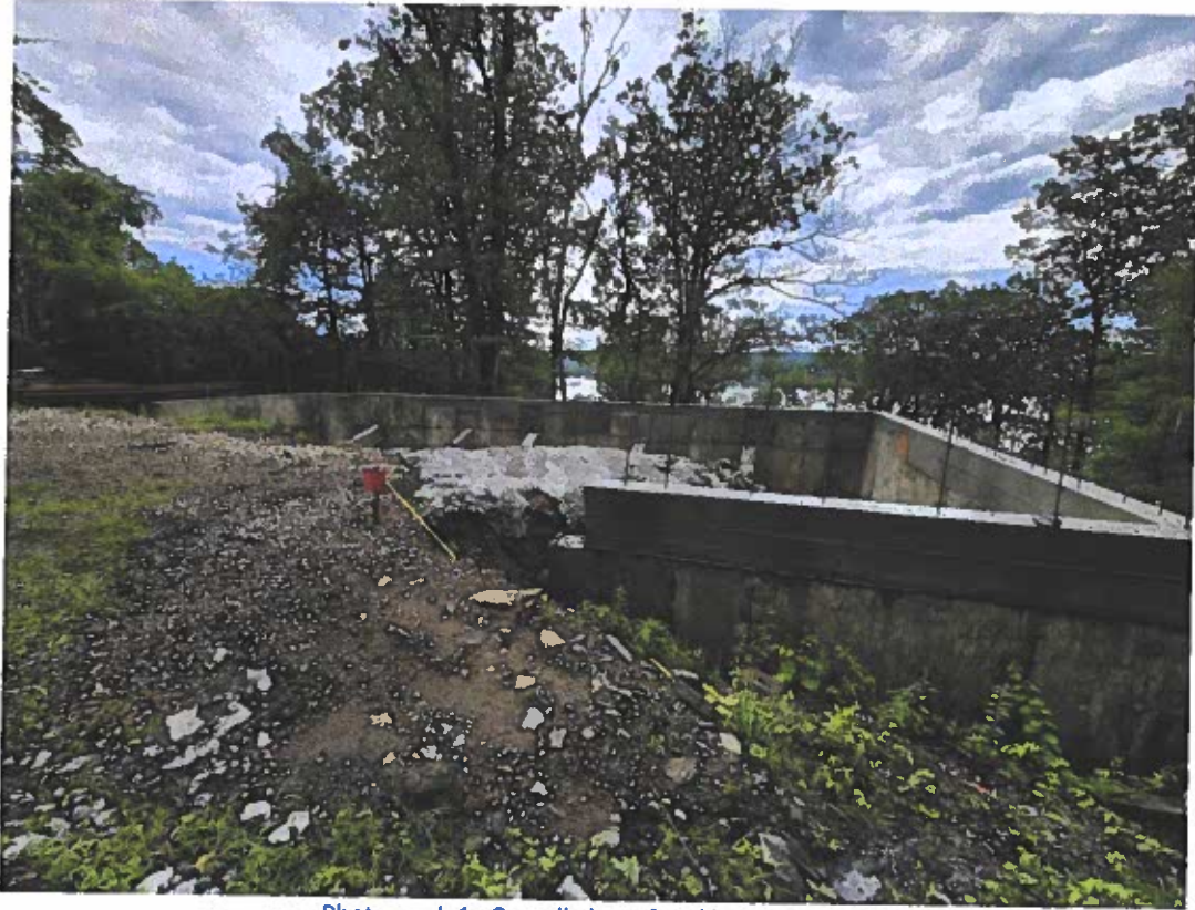
Photograph 1: Overall view of parking structure.
