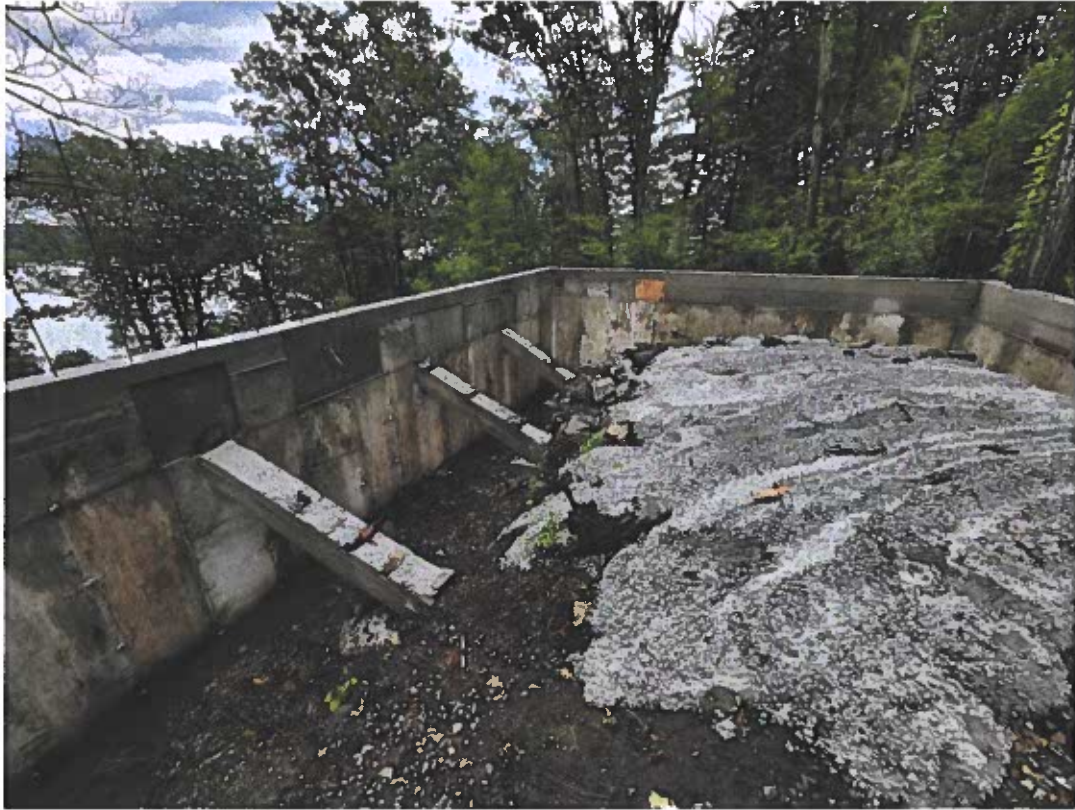
Photograph 2: Overall view of counter forts/butresses.
