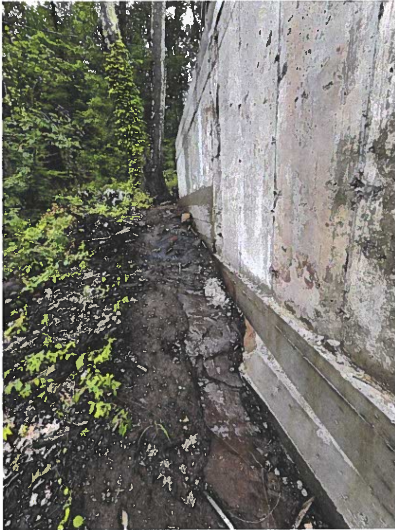
Photograph 3: Bedrock observed at stem wall casting.
