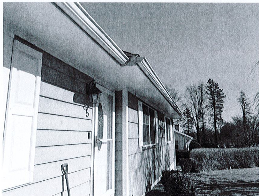
Existing Overhang at Front Door
