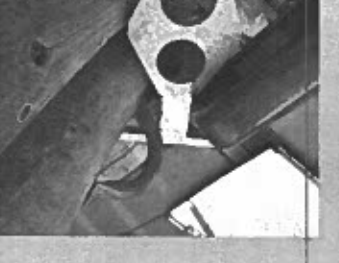
Partially Bound Opening Entrapment
